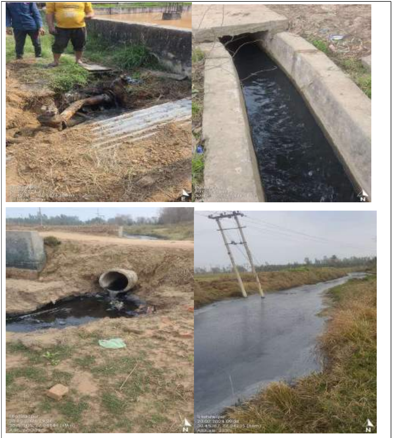
Photographs 22-25: Showing Bypass arrangement made by M/s Naraingarh Sugar Mills Ltd to discharge untreated effluent into the drain leading to river network:
